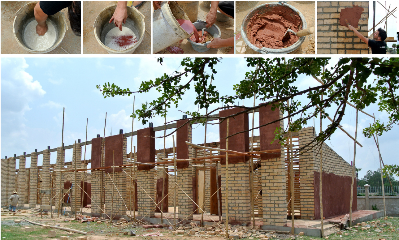
Fig. 8 Architeti senza Frontiere Italia, secondary school in Rong village, Cambodia. The construction phases highlight the use of raw earth block and natural plasters.
