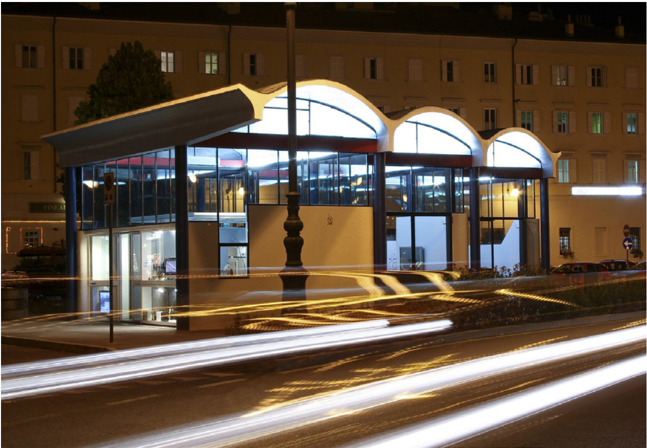
Fig. 1 Semerani e Tamaro Architet- ti Associati, Stazione Rogers, Restoration and Repurposing of the Aquila Company Service Station, Riva Grumula, Trieste, 2007-2008.
